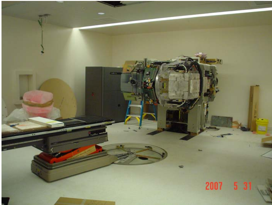
Linear Accelerator Installation in Progress
